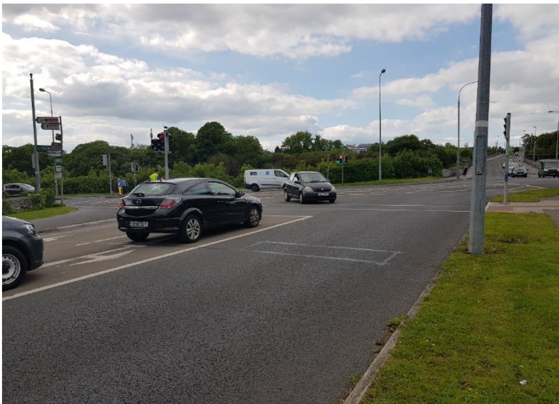
Figure 11.4: Existing Junction (Looking Northwards)
