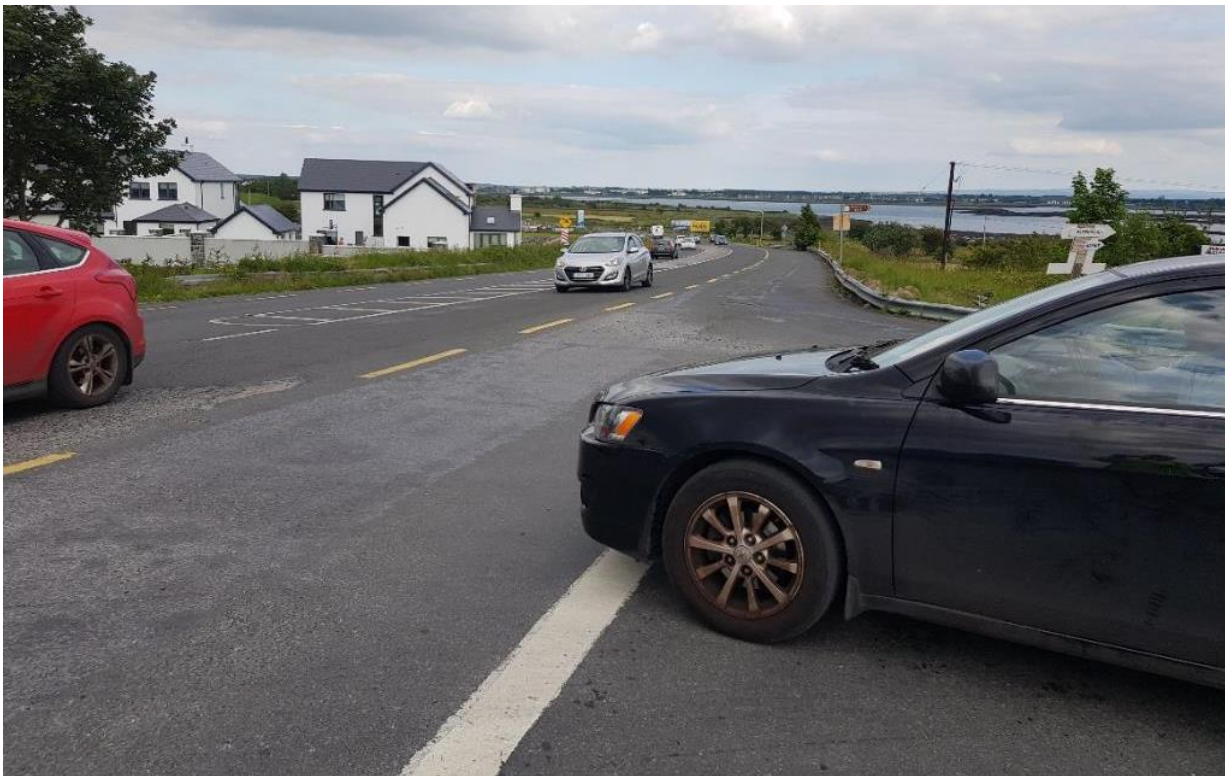
Figure 11.5: Existing Junction (Facing Eastwards)
